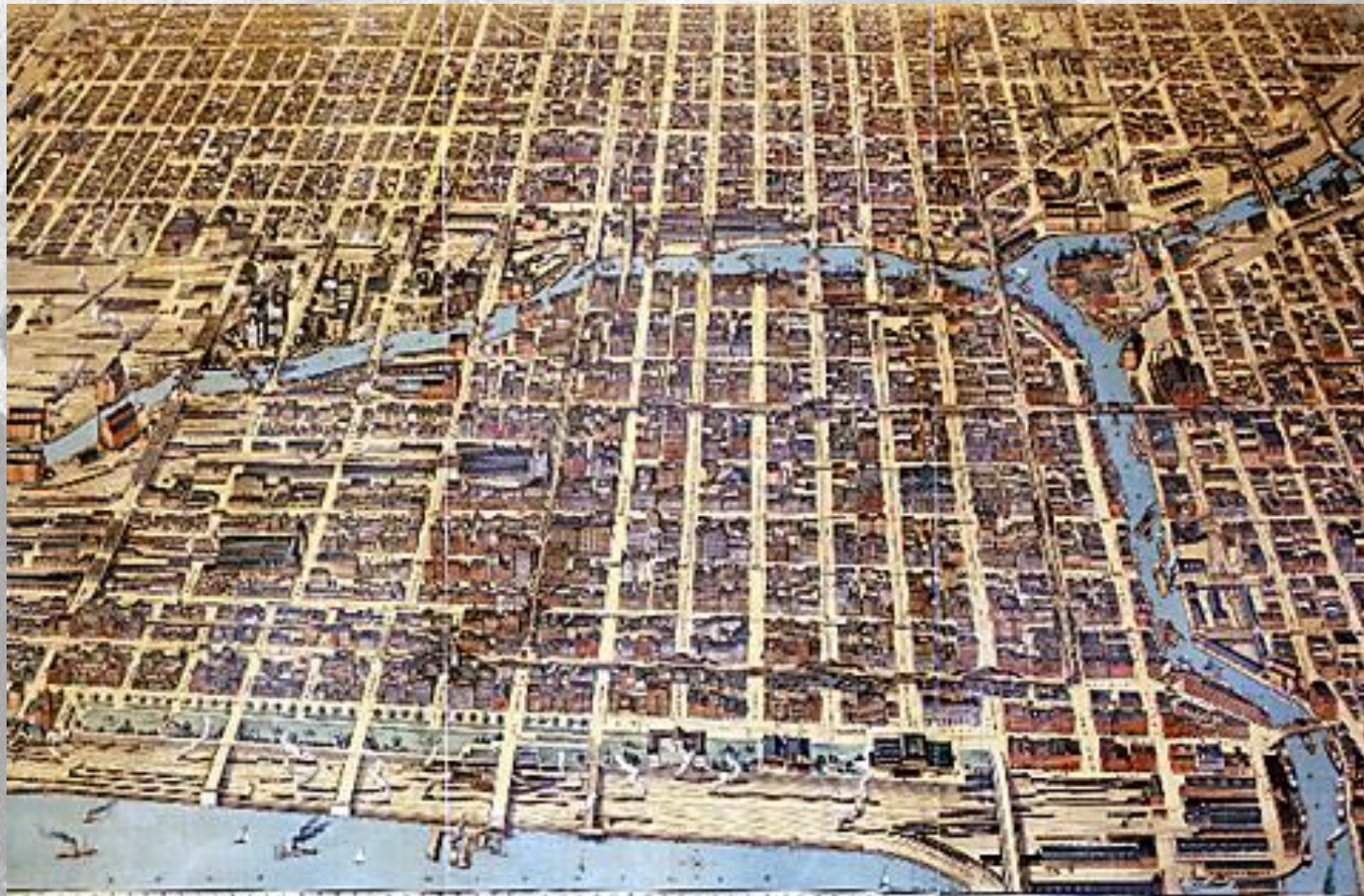
BIRD'S-EYE VIEW OF THE BUSINESS DISTRICT OF CHICAGO
